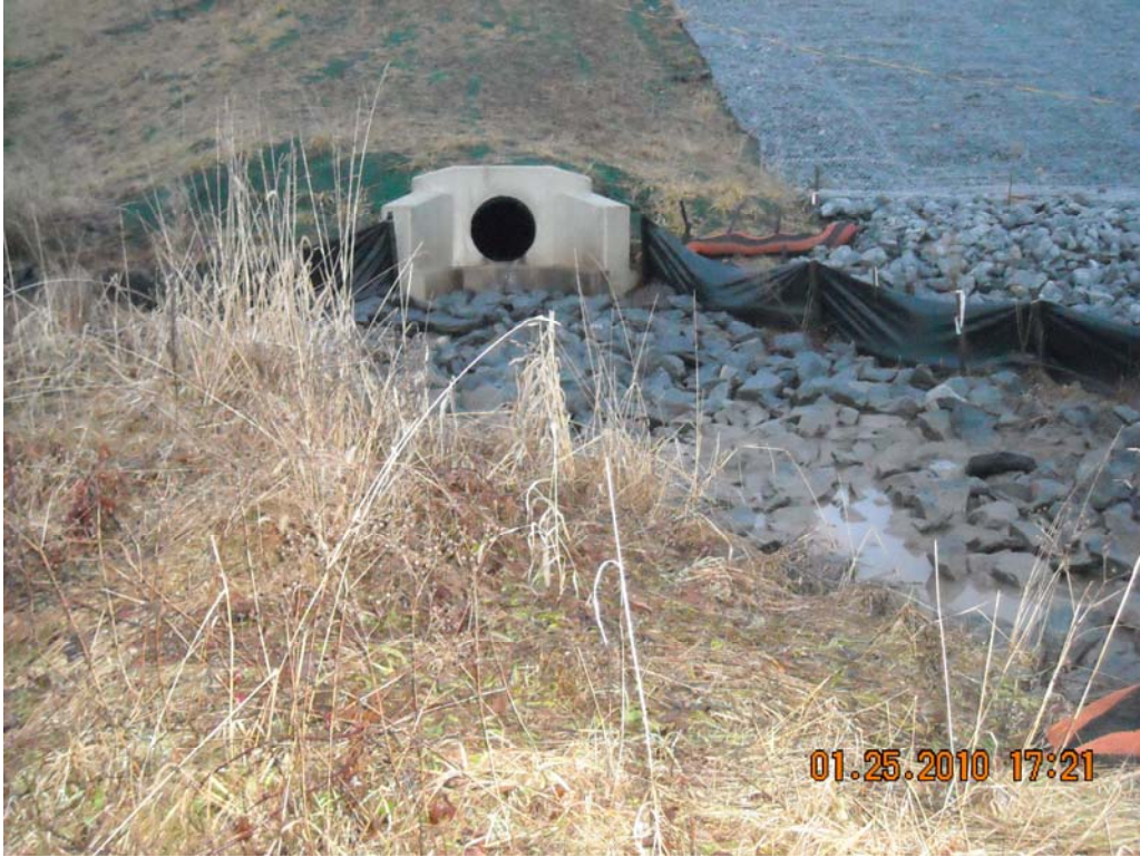
Basin discharge channel 01-25-10
