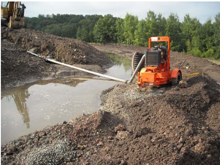
Picture 9: Pumping station set up at west end of CA
