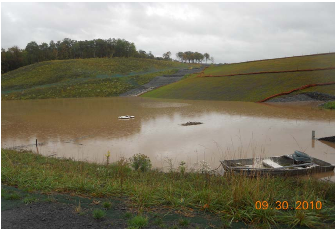
View of Sediment Basin on September 30, 2010 (facing northeast)
