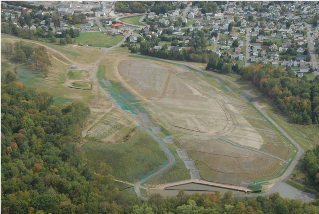
Aerial View of Site on September 28, 2010
