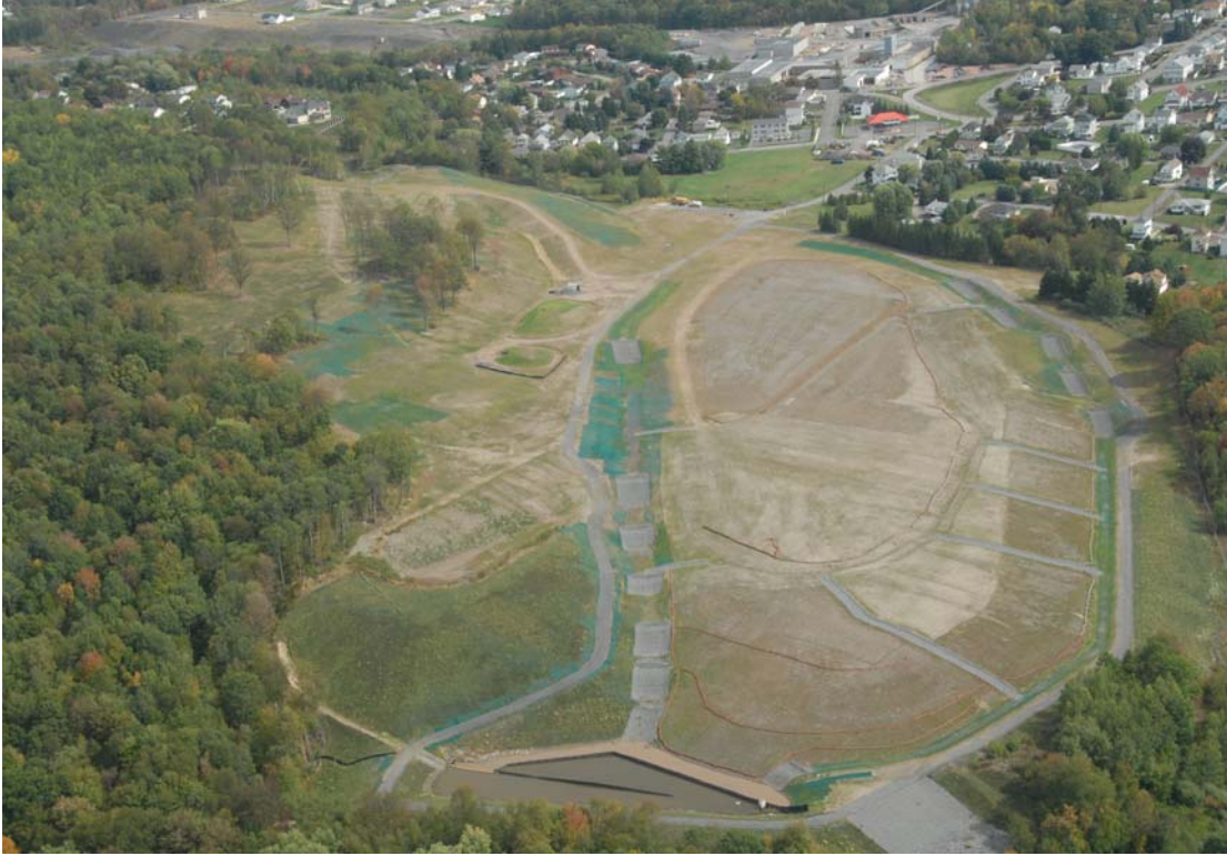
Aerial View of Site on September 28, 2010
