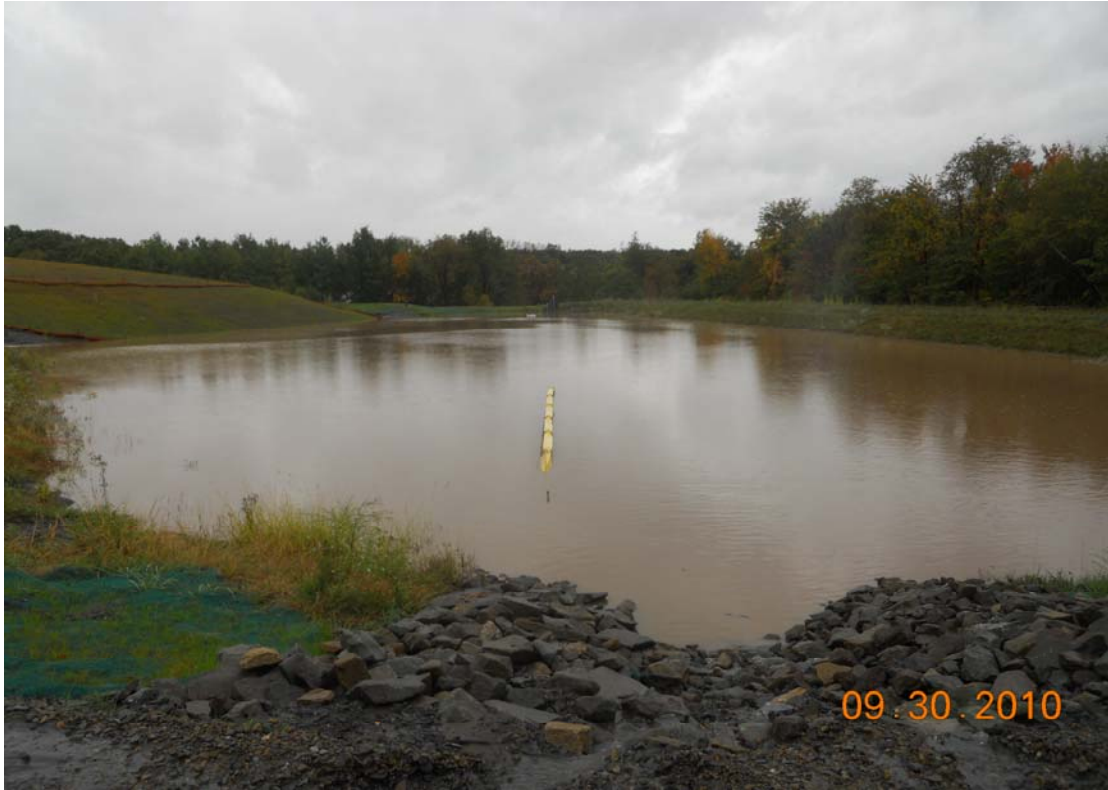
View of Sediment Basin on September 30, 2010 (toward Sulphur Creek)
