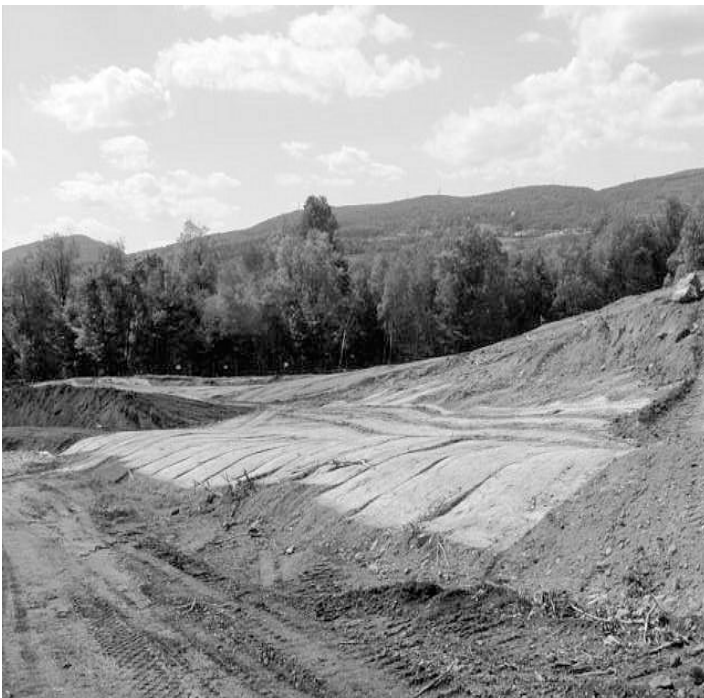
Construction of the New Stormwater Management Basin
