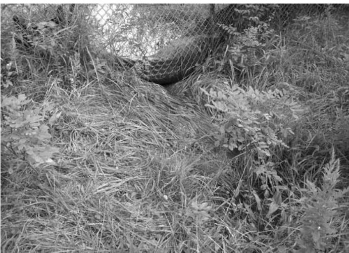
Discharge Point at Perimeter Fence
