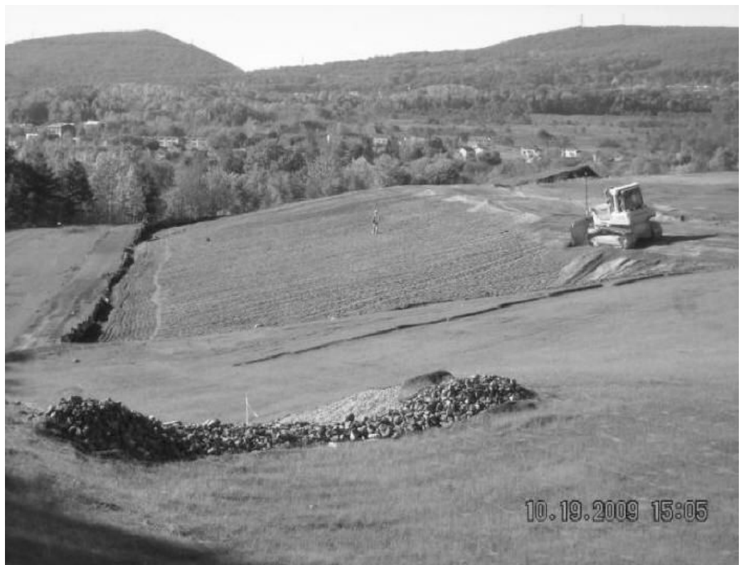
View of 4:1 Slope During Solidification Activities—10/19/09
