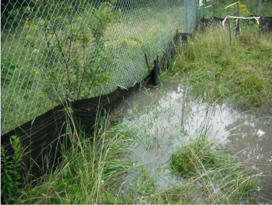
Picture 1: Discharge Channel Following CA Overflow (08-10-09)
